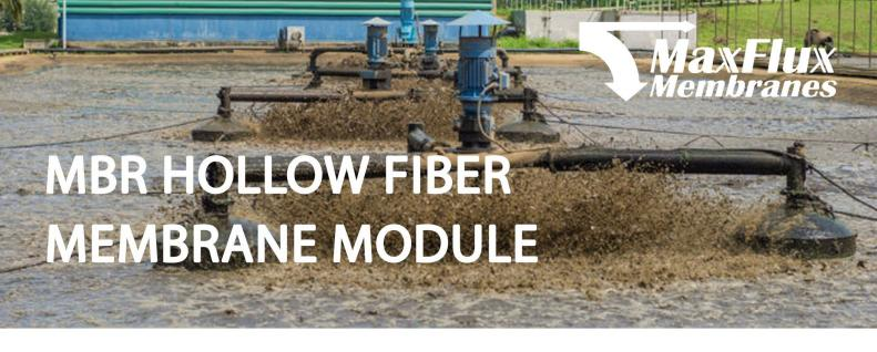
MaxFlux HF-MBR modules is an effective barrier against solids, bacteria to be separated from water and turn the wastewater into a viable water source. MaxFlux hollow fiber MBR membrane is made of reinforced PVDF which is produced through Thermally Induced Phase Separation (TIPS) with the PET inner-support material Comparison to the normal PVDF hollow fiber membranes it has a higher strength stronger anti-peeling condition, higher porosity, and larger flux
